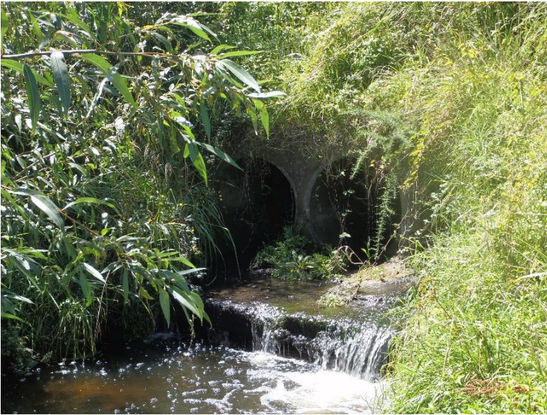
Figure 2: Awarua Stream fish passage restoration by culvert replacement. Photo on the left taken in 2013 and the right in December 2019 after replacement of the culvert and installation of a leaky weir downstream of the culvert.
